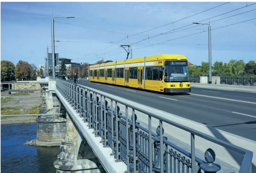
← The reconstructed Albertbrücke
