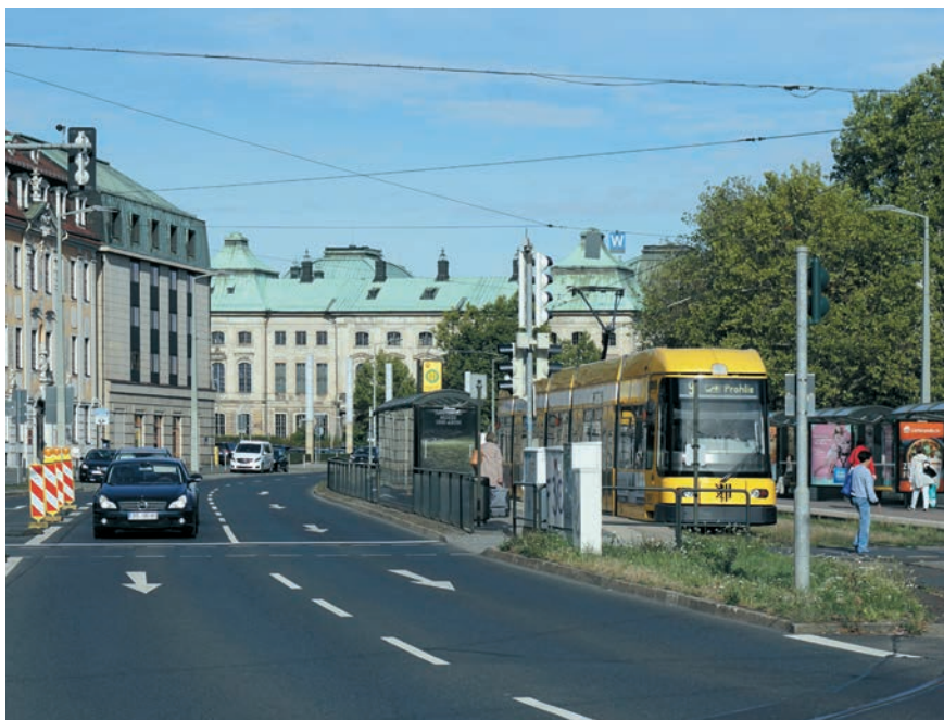
↓ Große Meissner Strasse, view to the north-west
